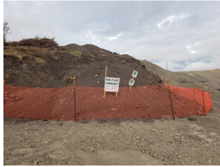
Sept 12/18 Photo facing North West SF 35 (KP967) Rare plant material fenced off and kept separate from other soil piles.
