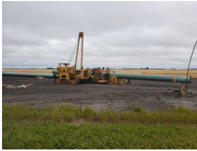
Sept 12/18 Photo facing North SF 24 North side of the road Pipe bending taking place.
