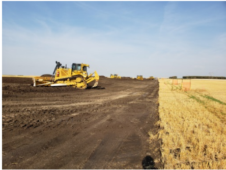
Sept 11/18 Photo facing West SF 44A KP 986+746 Dozers stripping the ROW
