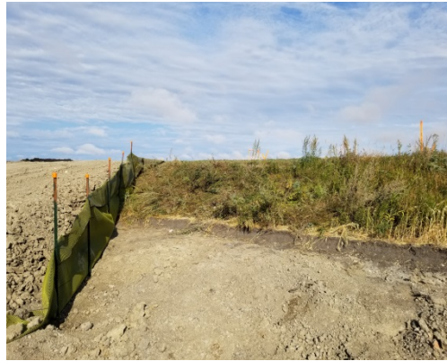
Sept 12/18 SF45 Facing West. Silt fence and cutting of edges.
