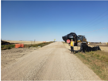
Sept 10/18 Photo facing West SF 43 Access Excavator crossing road with flaggers in place
