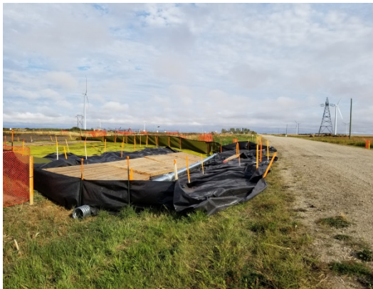
Sept 12/18 SF47 facing North. Silt fence geo- tec and pads laid down for approach to be covered.
