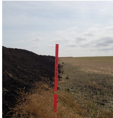
Sept 11/18 Photo facing East SF 44 (Between KP983+300 and KP 983+500) View of top soil exceeding the limit.
