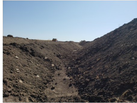
Sept 10/18 Photo facing east SF 44 (KP984+923) View of top soil and seconds piles.
