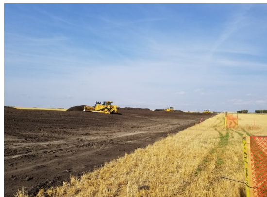
Sept 11/18 SF 44 Cats piling topsoil
