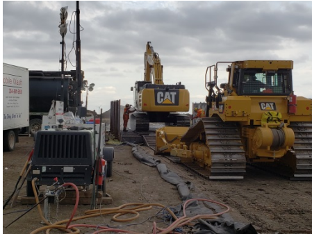
Sept 11/18 Photo facing East SF 44A cleaning station Excavator being cleaned by compressed air and water
