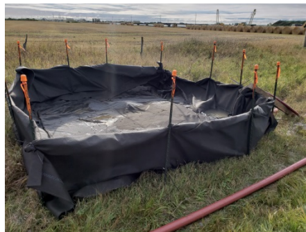
Sept 12/18 Photo facing South East SF 19 (KP936+720) Water being pumped into Geo bag.
