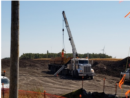
Sept 10/18 Photo facing South East SF 45 East side of the road Semi unloading access mats
